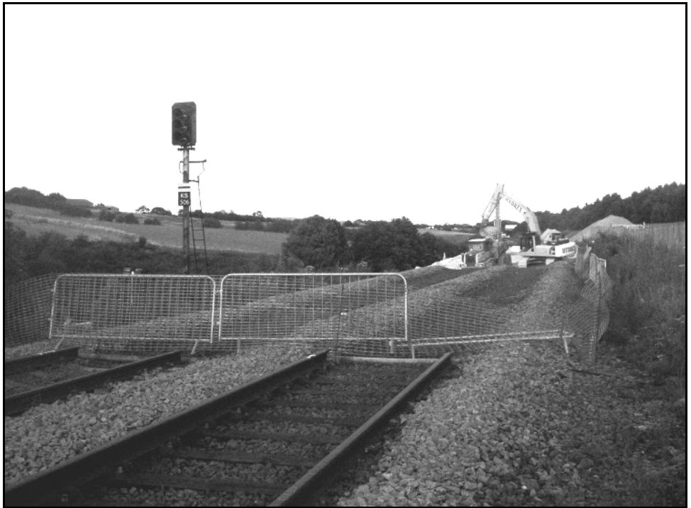
Waleswood on the Sheffield-Worksop line on 30 July 2007. Flood damage closed the line on 25 June and work is being carried out to reconstruct the embankment using aggregate instead of spoil. An aerial view, taken by Chris Booth, of the damage caused can be found on p77 of the September issue of The Railway Magazine.
