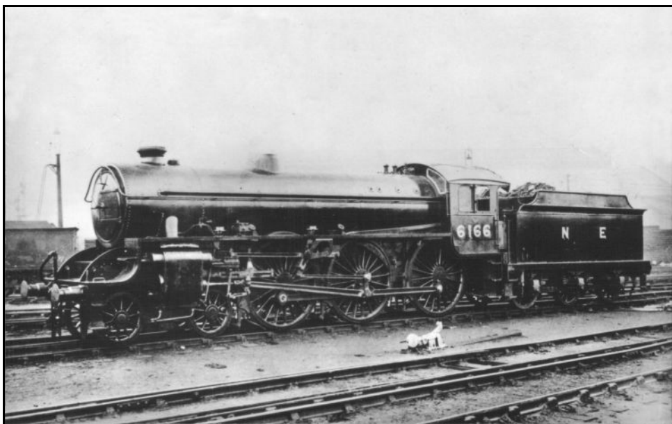
LNER class B3/3 4-6-0 no.6166 after rebuilding by Thompson in 1943. photo : GCRS Collection
